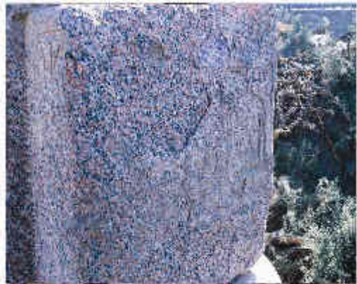
Fig. 8: Scaling is observed on granites.
