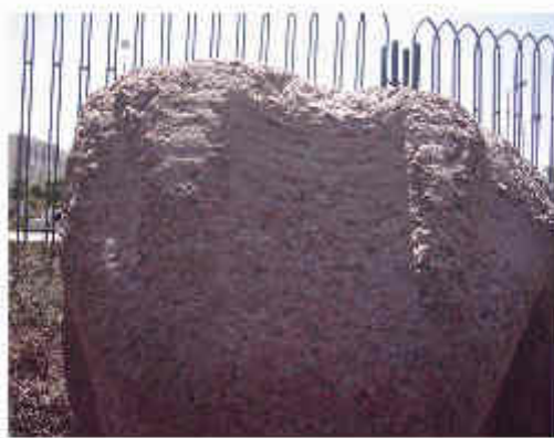
Fig. 9B: Loss of details in granite statues.
