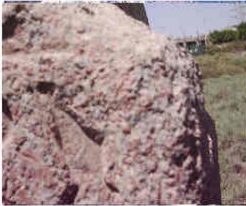
Fig. 7A: Granular disintegration is grain by grain disaggregation .
