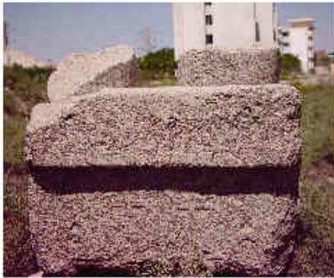
Fig. 7C: Granular disintegration is grain by grain disaggregation.
