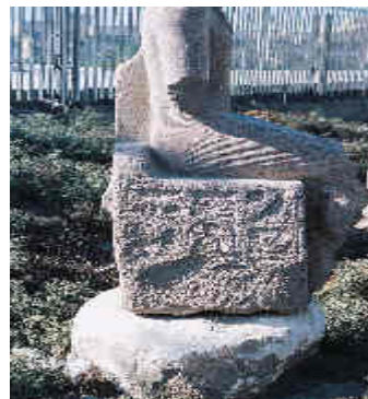
Fig. 5: Biocolonization, plant roots grow in the fractures of granite statues.
