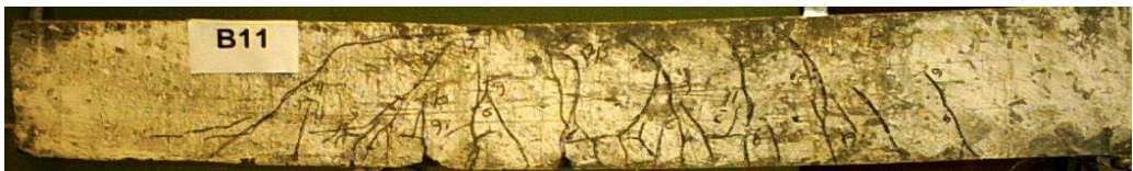
Fig. 2.e: Pattern of crack of the tested beam (B11).
