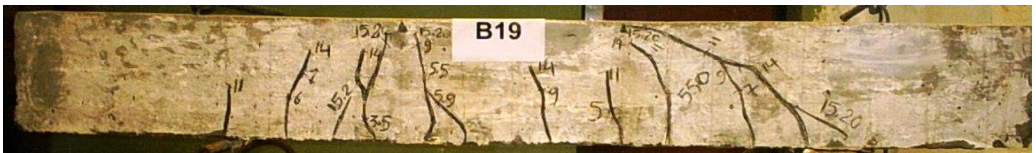
Fig. 2.k: Pattern of crack of the tested beam (B19).
