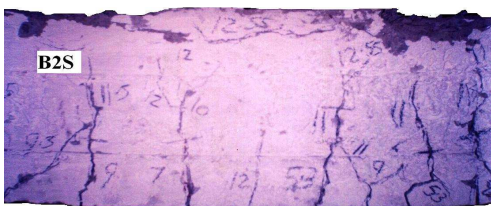
Fig. 6e: Failure shape of beam (B2S).
