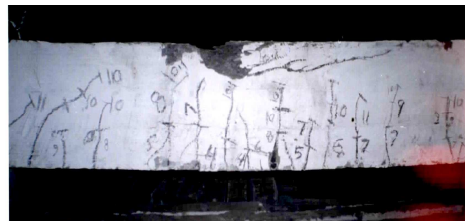
Fig.5b: Failure shape of beam (B2).
