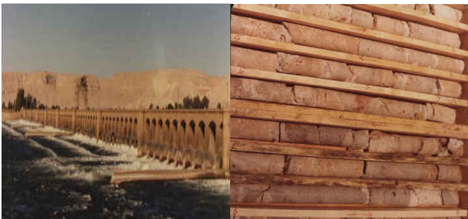
Fig. 1: The barrage and samples.
