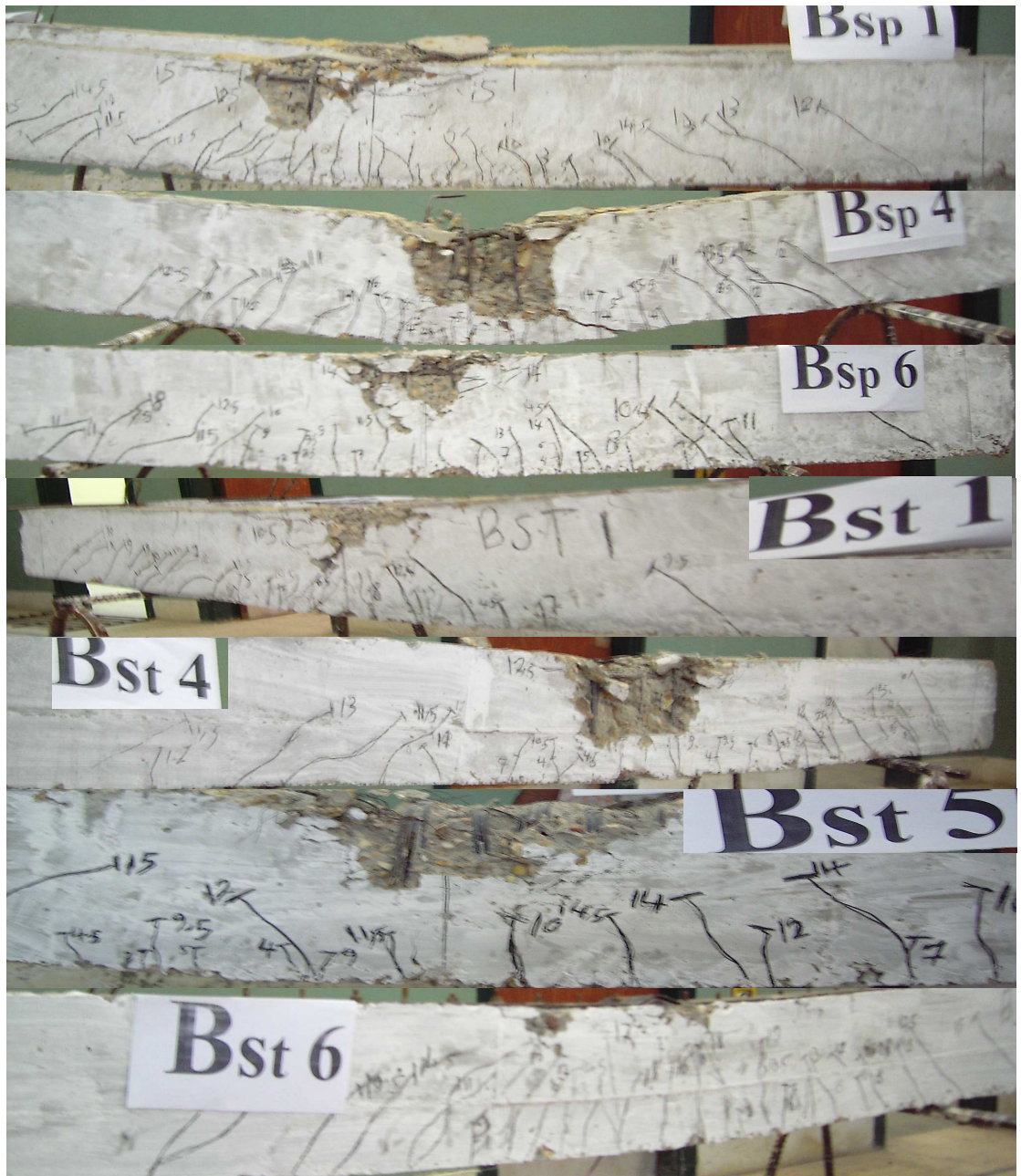
Fig (12):Pattern of cracks and modes of failure for tested beams.
