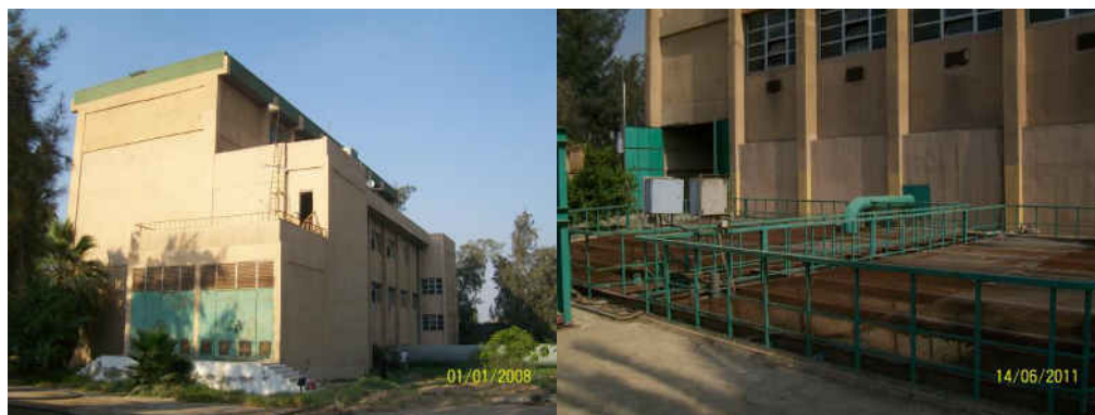
b) Pumping station building from outside
