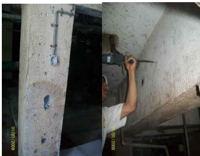
Fig. 8 Compression test specimens taken from structural elements.
