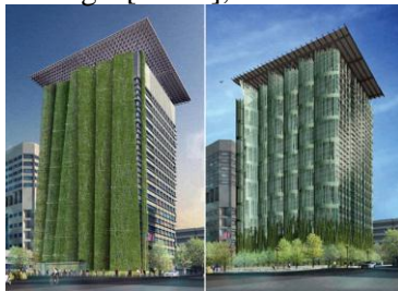
Fig. 9. The living wall in the original design (left) for the Building has been replaced with a system of aluminum rods (right) [38]
