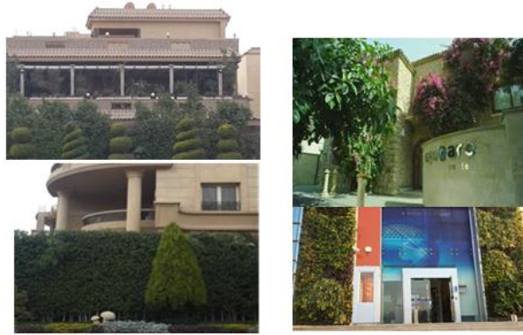
Fig. 11. Randomly selected buildings showing balcony planting, container system, and direct green screens especially cable system. Cairo. [Source – Researcher]
