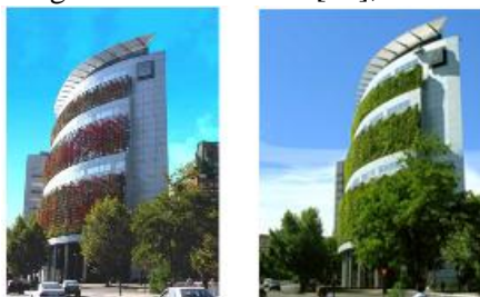
Fig. 8. Colorful facade at autumn (left), Green facade at summer (right) [36]
