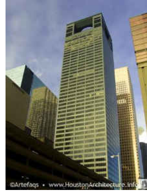
Center Point Energy Plaza, Houston, Texas, JV III , 1973 [23] .
