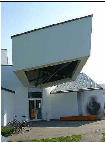
Vitra Fire Station, Weil am Rhein, Germany, Zaha Hadid, 1989-93 [20].
