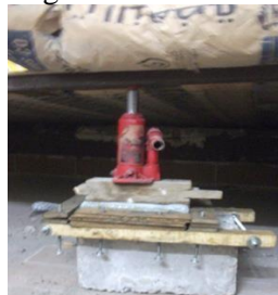
Fig (2-4): Pressure done using a hydraulic jack.
