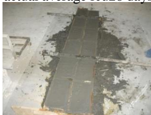
Fig (2-1): Molding of concrete prisms
