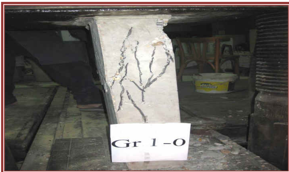
Failure mode, (unconfined rectangular R.C. columns) ( FM 1)
