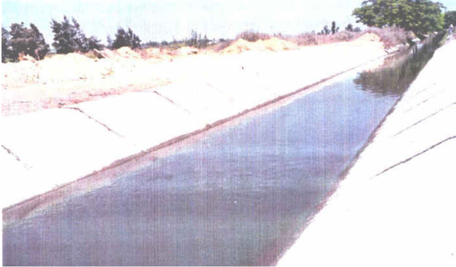
Fig. 9. The innovative lining applied to a canal reach
