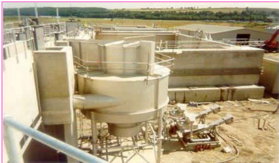
Fig.1. Configuration of hydrodynamic separator
