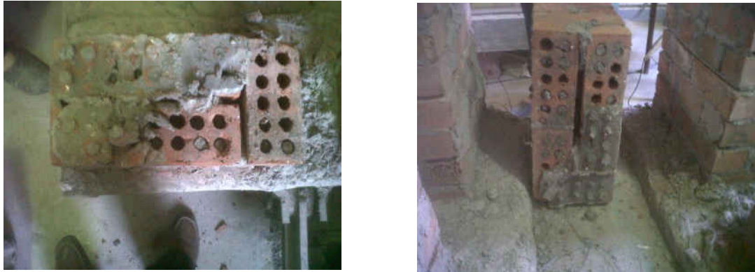
Fig. 16. Typical crack surfaces for failed piers.
