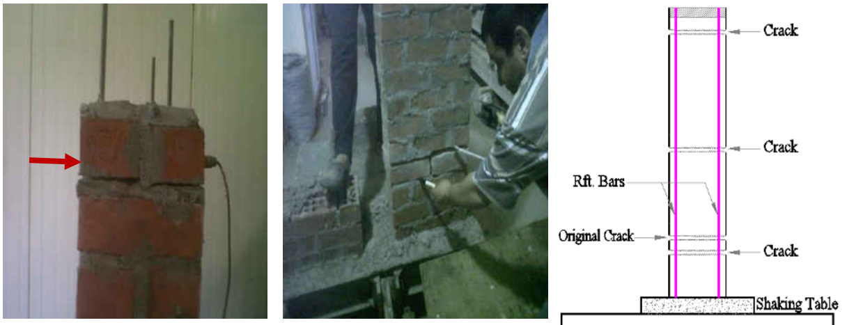
Fig. 14. Failure pattern for stapled piers.
