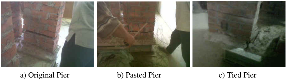
Fig. 13. Failure pattern for repaired piers.
