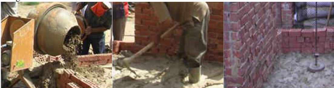
Fig. 15. Backfill with soil mixes with cement dust
