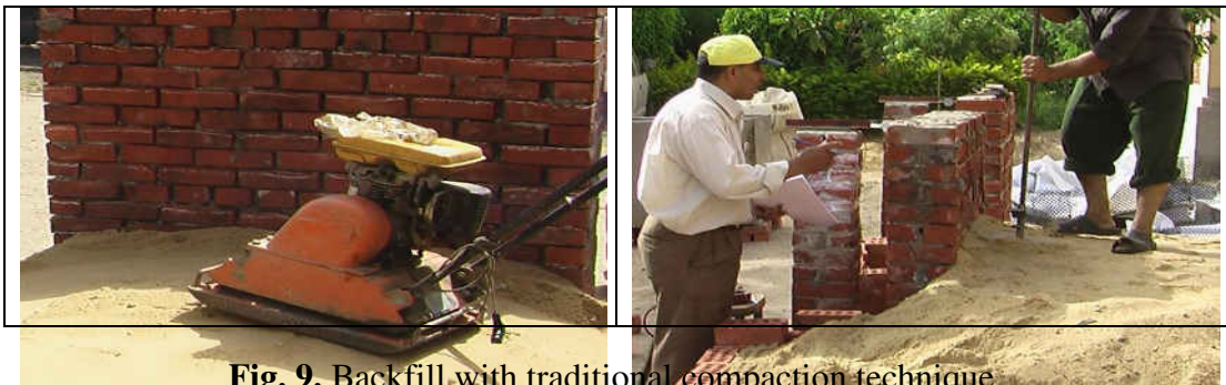
Fig. 9. Backfill with traditional compaction technique.
