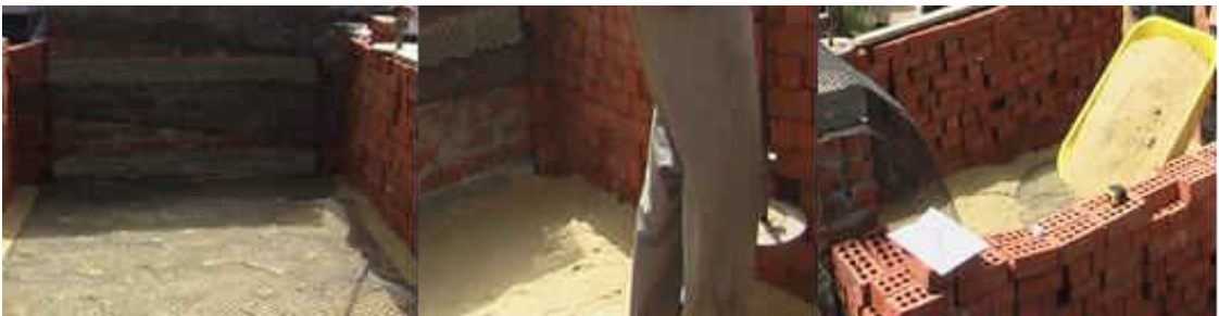
Fig.11. Backfill with geogrid reinforced soil
