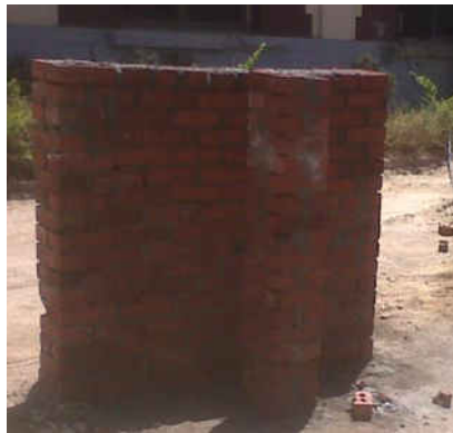
One of the tested wall
