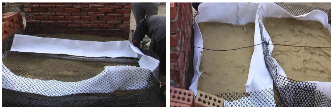
Fig.13. Backfill with gabions boxes filled with sand
