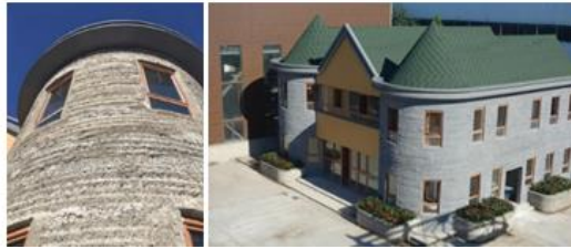
Fig. 3. The 3D Printed villa onsite. Source: [23]
