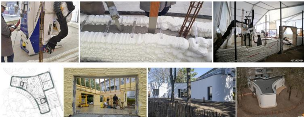
Fig. 5. Robotic 3D Printed YHNOVA House: plan of Yhnova™, different views. Source: [34, 35]
