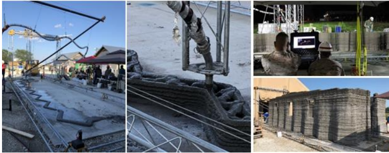
Fig. 7. the construction site of US Army barracks, Champaign, Illinois. Source: [41, 43, 44]
