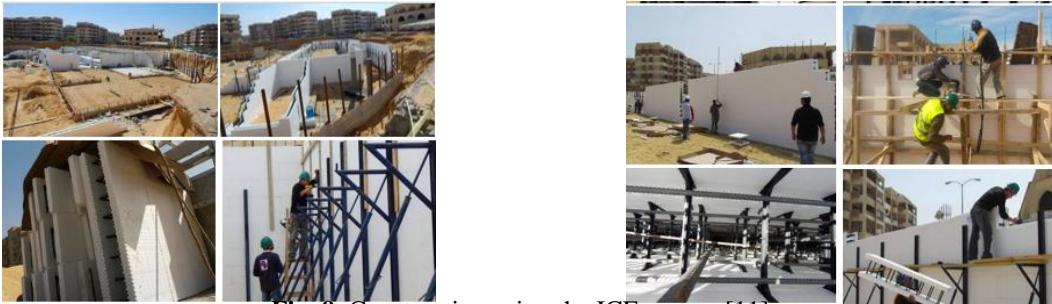
Fig. 9. Construction using the ICF system [11]
