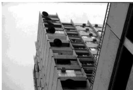
Fig. 34. Satellite dishes hanged on facade
