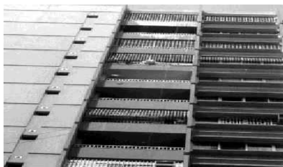
Converting balconies into interior spaces
