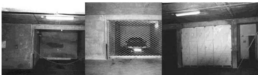
Fig. 44. Placing a chain or installing a door by residents for security of the car parking spaces
