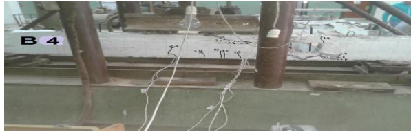
Photo 7. Crack pattern of beam "B4".
