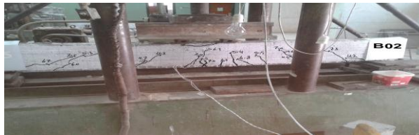
Photo 3. Crack pattern of beam "B02".
