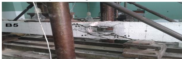
Photo 8. Crack pattern of beam "B5".
