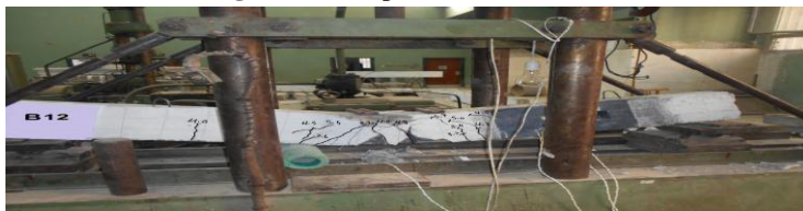
Photo 15. Crack pattern of beam "B12".
