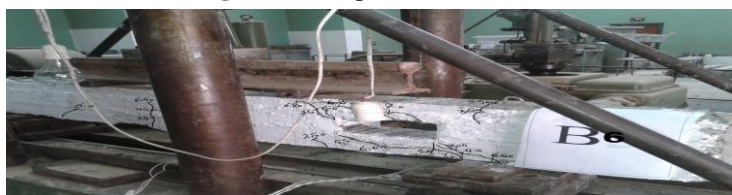
Photo 9. Crack pattern of beam "B6".
