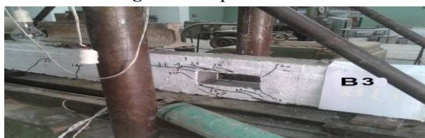
Photo 6. Crack pattern of beam "B3".
