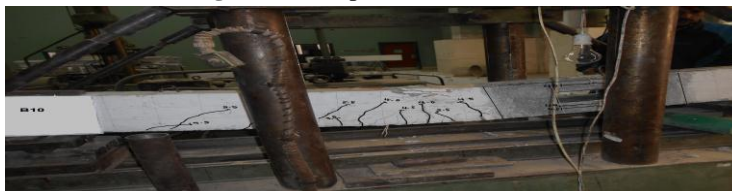
Photo 13. Crack pattern of beam "B10".
