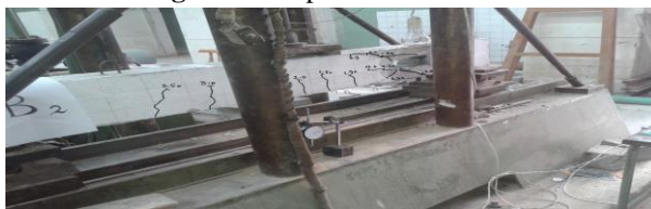
Photo 5. Crack pattern of beam "B2".
