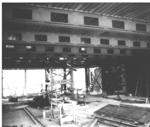
b. Rectangular opening for building facilities.
