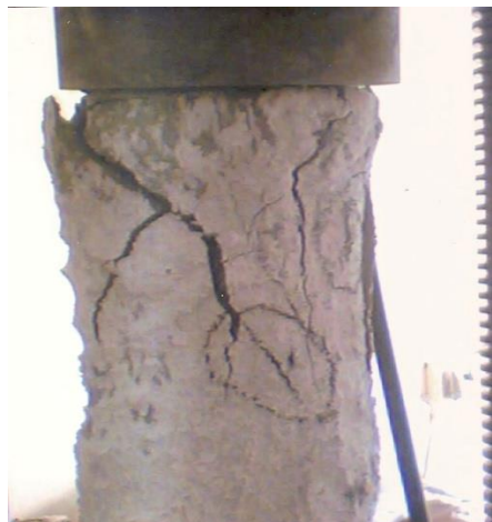
Figure (13) Cracking of circular column and the .The cover stated to spall out.
