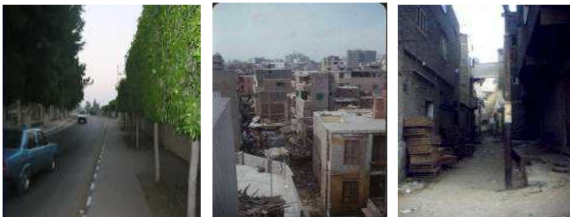
Photo2: deteriorated Residential areas inside Mansoura City
