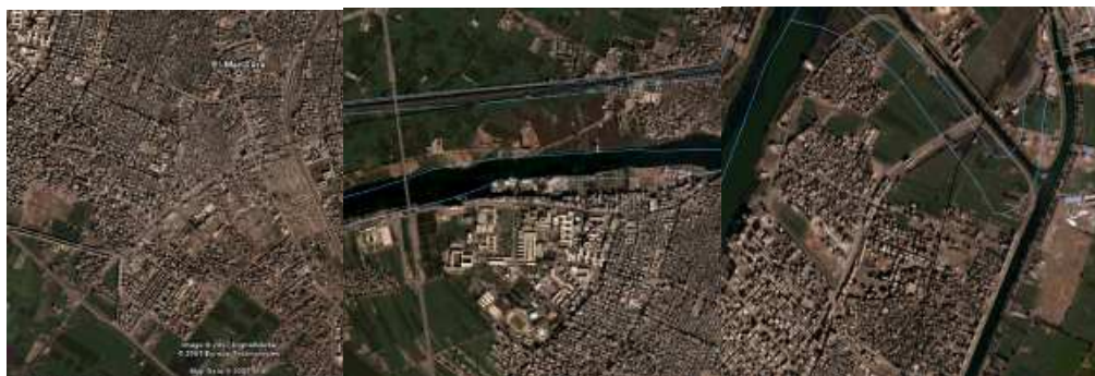
rural pockets in south part rural pockets in west part rural pockets in east part
