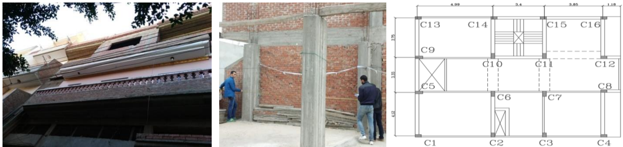
Fig 10 Building (II) Photo during field study and showing its floor structural system
