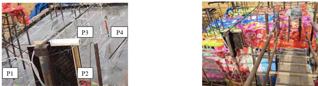
Figure 7: Curing method of plastic film and quilt
