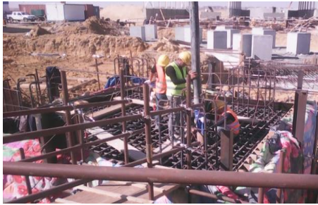
Figure 2: Raft reinforcement
