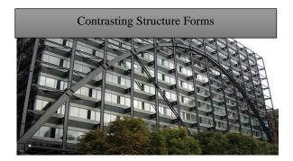
Fig. 10: Exchange House, London, England, Skidmore, Owings & Merrill, 1993. Showing Arches enable the building to span the site. Source: [3].
