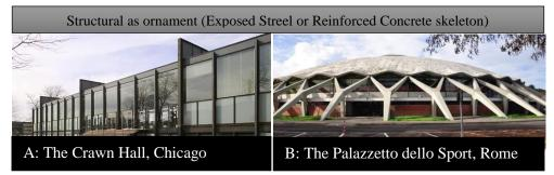
Fig. 4: A) The exposed steel skeleton, including the plate girders that rise above the roof was used as source of ornamentation in the Crawn Hall, Chicago, USA, 1952-56, by Mies Van Der Rohe. B) The exposed inclined exterior reinforced concrete struts were used as source of ornamentation in the Palazzetto dello Sport, Rome, 1957, by Anni bale Vitellozzi, Source: A: [3]; B: [42] respectively.
