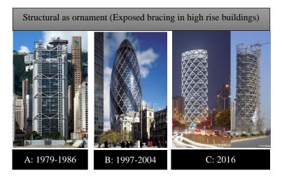
Figure 5: Different forms of the steel bracing in high rise buildings, used as a source of ornamentation. Source: A:[22]; B:[23]; C:[24]
