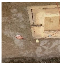
a) The location of the thermal sensor on wall
