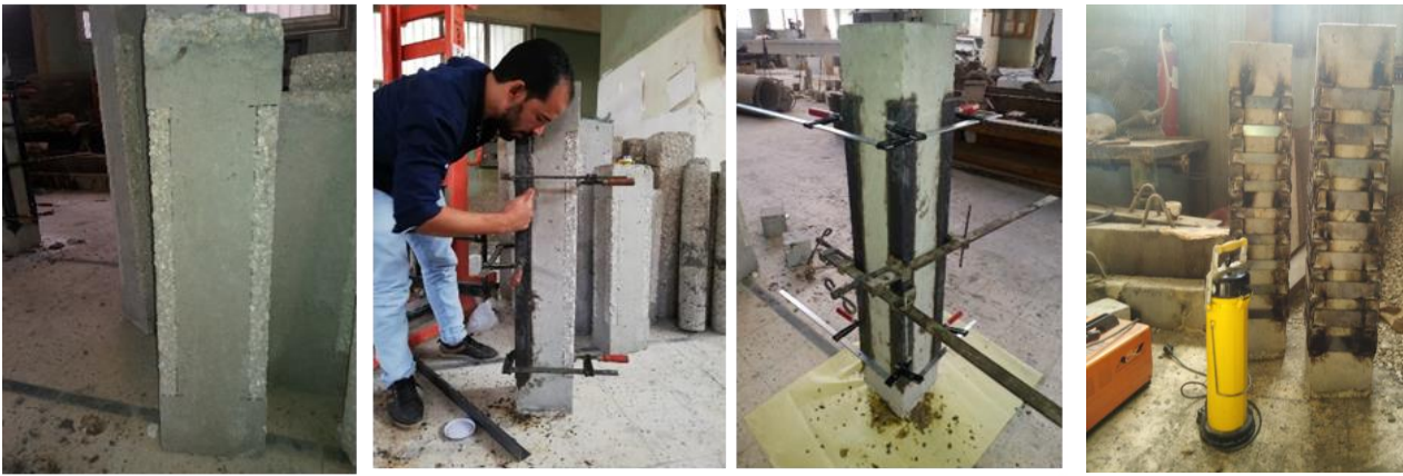
Fig. 2: Preparing concrete surface and steel jacket application.
