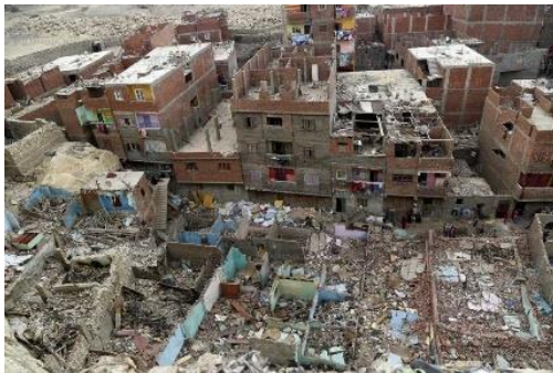
Fig. 2: El-Deweka before rehabilitation
