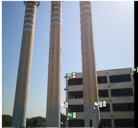
Fig. 2: Distribution of control points on the studied chimney and neighboring elements.
