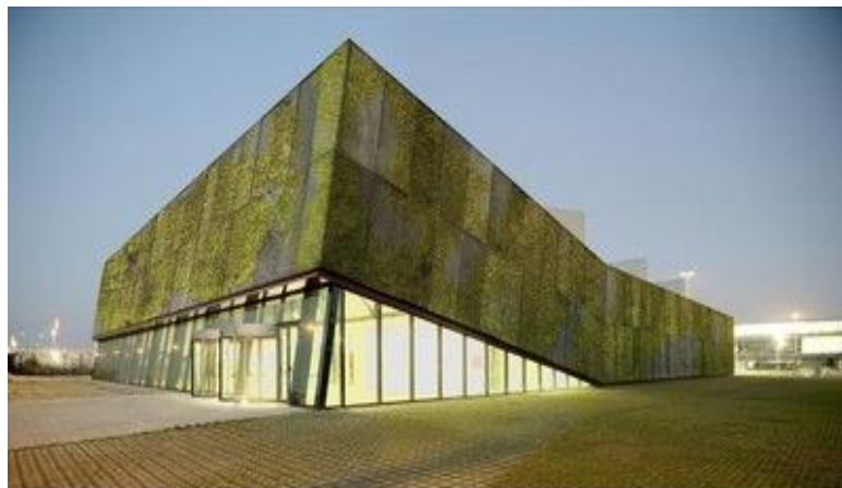
Figure 7. Biological concrete to create green facades for the Aviation Cultural Center 41
