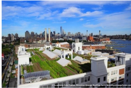
Fig.13:"The Brooklyn Grange" project in New York City [30]
