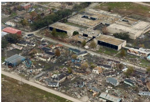
Fig.19: General site condition of the school before the project began[35]
