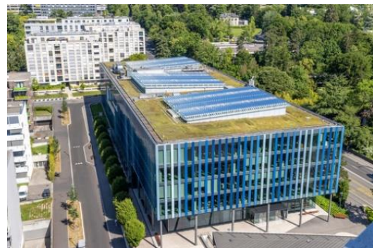
Fig.25: Final shape of one of the rooftops after completion [41]
