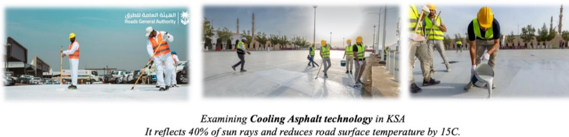
Figure 9: Saudi Arabia's implementation of the experiment “Cooling Asphalt Technology” [65]
